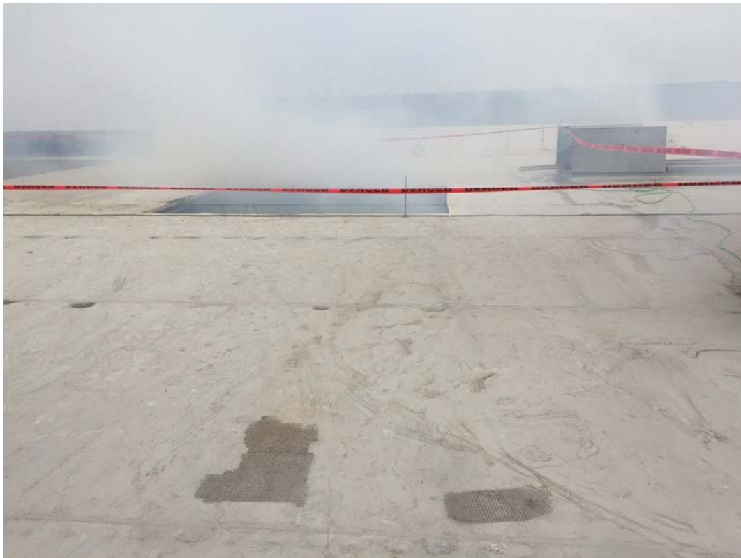
Figure 10 Ventilation hatches open and roof opening by Centimark (December 12, 2016)
