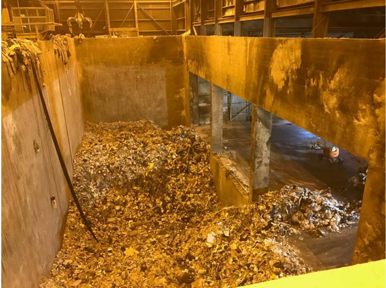
Figure 4 Refuse Pit and Tipping Floor (01/18/2017)
