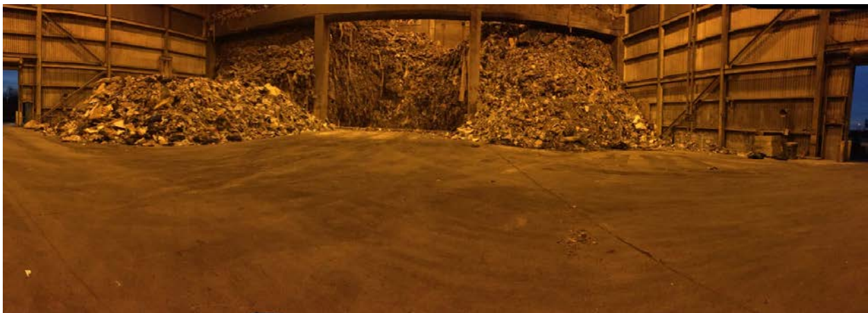
Figure 5 Refuse Pit and Tipping Floor (12/05/16)
