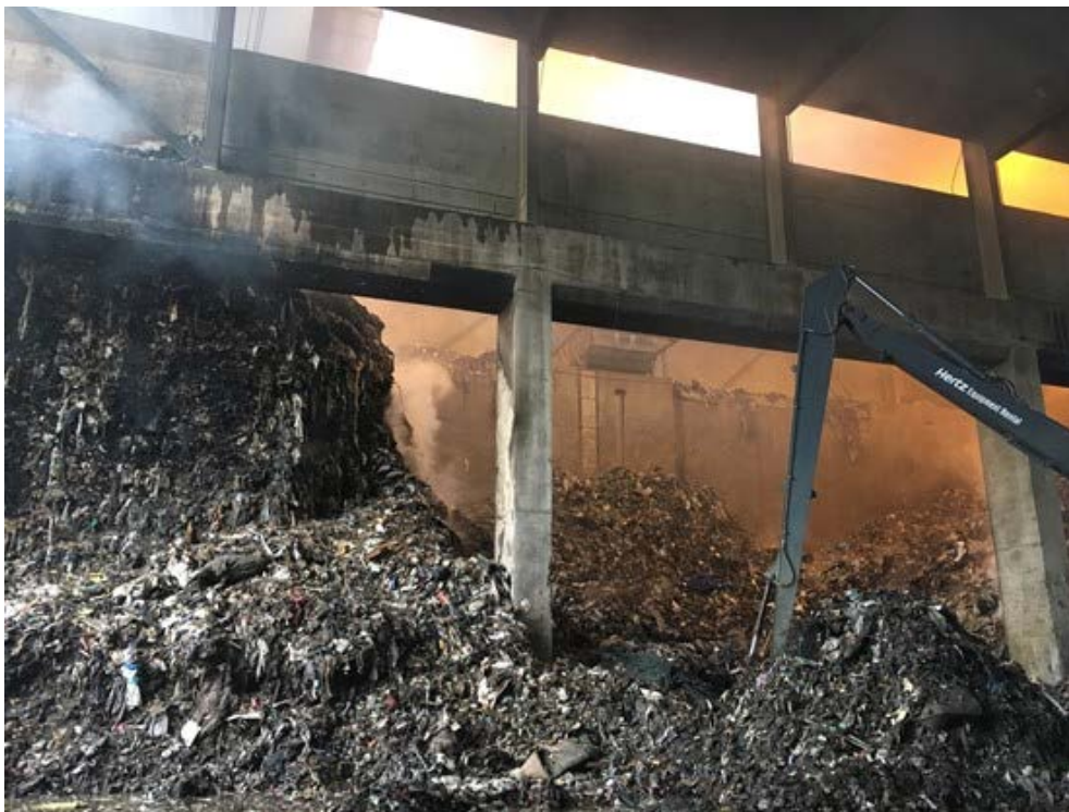
Figure 7 Trash level up to 85 foot mark in Bay A (12/10/16)
