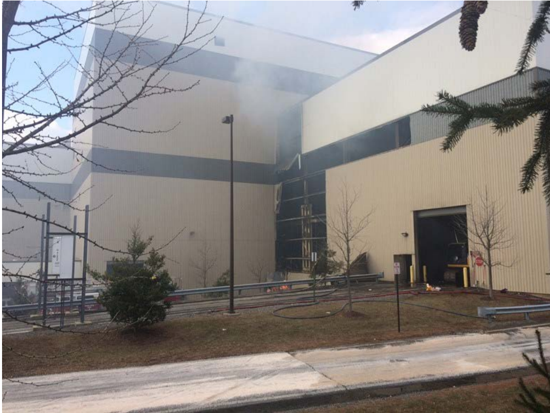
Figure 9 South wall horizontal ventilation openings (12-10-2016)
